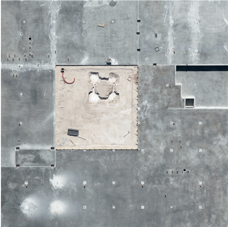
Construction site, Stains, 2019
