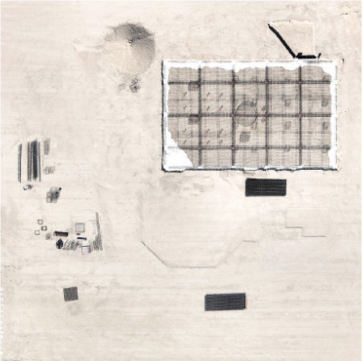
Construction site, Achères, 2012
